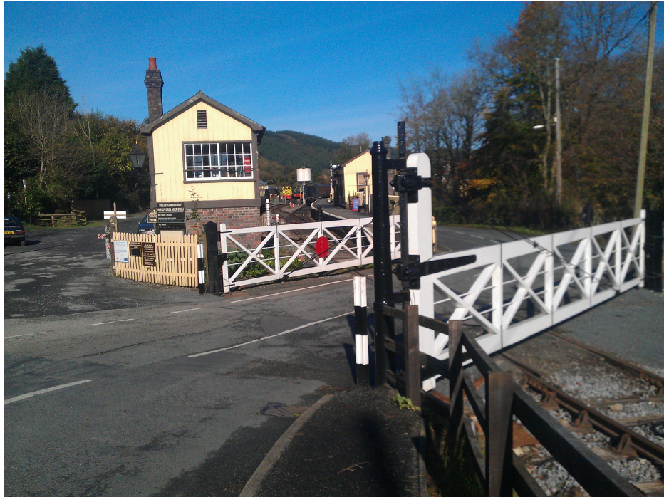
Figure 11.2: Terminal view of Bronwydd Arms Station. From the level crossing to behind the camera's view is the beginning of the new line.
