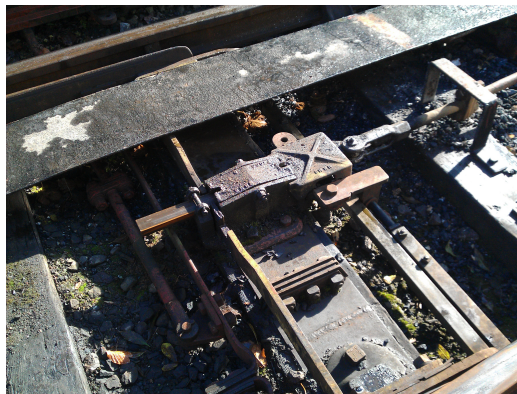
Figure 11.9: Facing-point lock is clearly visible in centre of image, the bar parallel to the tracks slides back and forth to lock/unlock the set of points. The bar orthogonal to the track is called the stretcher bar, and has two cutouts (one for normal and one for reverse position) that the first bar will slide into/out of.
