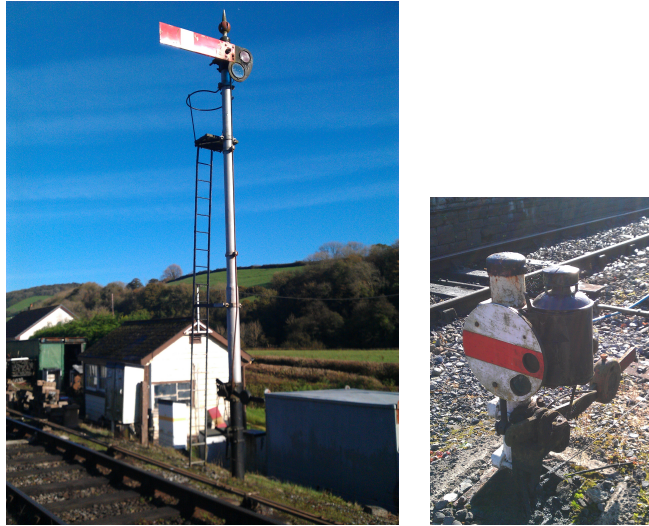
Figure 11.8: Different types of signals in use, left is a semaphore signal (19) and right is a shunting signal (17).
